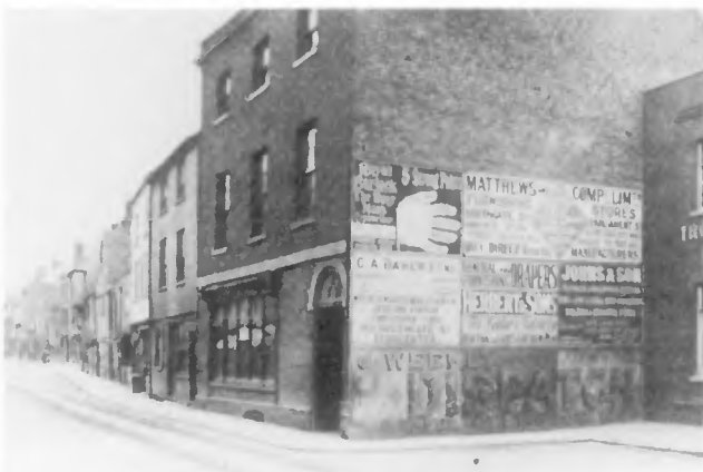
Plate 4. A view of Westgate Street 1902, taken just west of where Foreign Bridge formerly stood, which is now deeply buried. These buildings to Lower Quay St. were demolished c. 1907 for road widening. From the Gloucestershire Collection.
