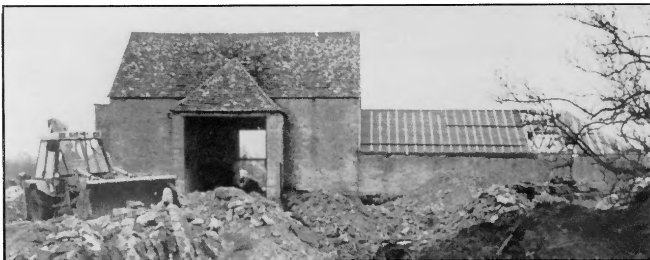
Barn conversion in progress
