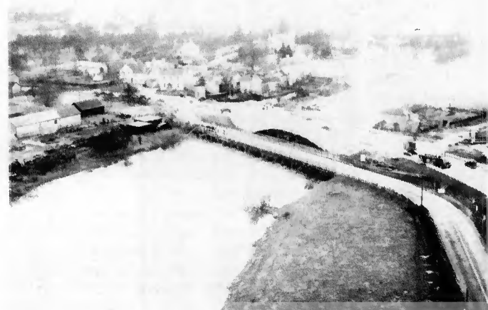
Maisemore bridge under construction, early 1950s.
