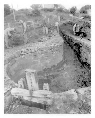
Fig 5. Cutsdean sheepwash being repaired
