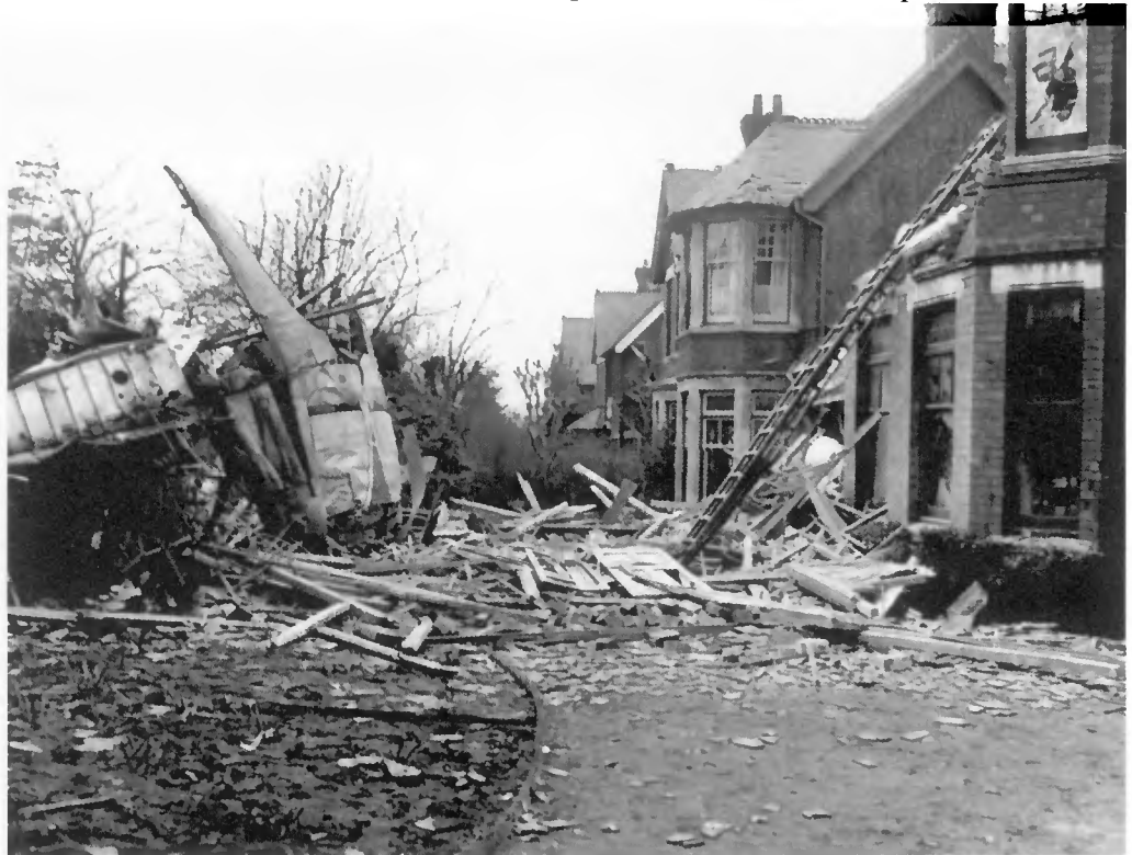
Fig 4. The port engine and debris from the impact fill Longmead's front garden.
